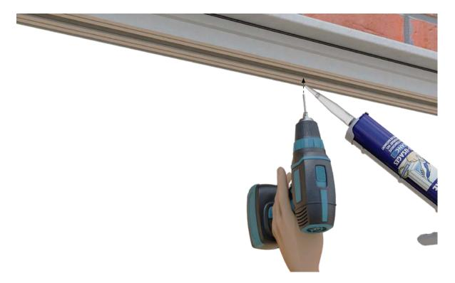
16 Insert suitable sealant to fixing hole, then screw preferred fixing in place. Repeat process along the bottom track, ensuring fixings are within 900 mm intervals.
