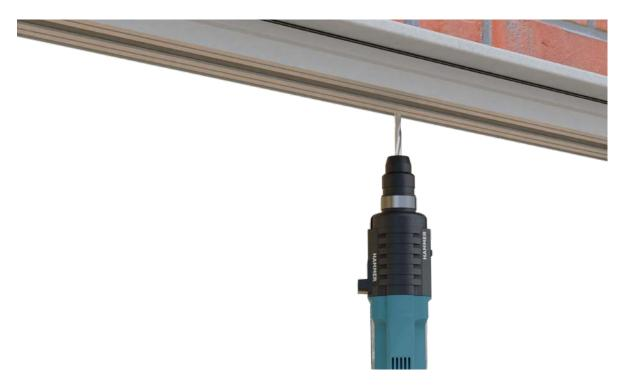
Drill and countersink an appropriate sized fixing hole through the frame. This should be no more than 200 mm from the external corner of the frame.
